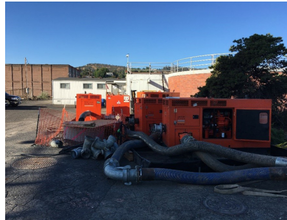
A total of five diesel self-priming pumps were used to handle peak flow events and prevent a sewage spill during the influent pump station retrofit.
