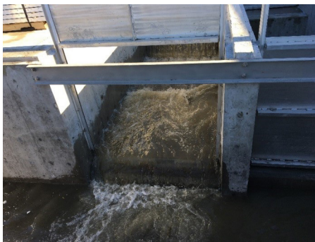
Critical flow split at the primary filters promotes secondary process stability.
