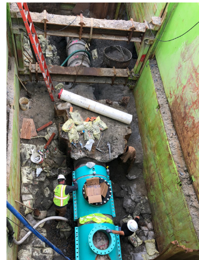
The excavation at the beach was protected from tidal influences so that reconnection to the existing outfall could be completed.
