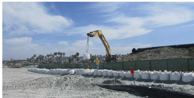
The contractor elected to construct a sandbag platform backfilled with sand to elevate the work area above the high tide line.
